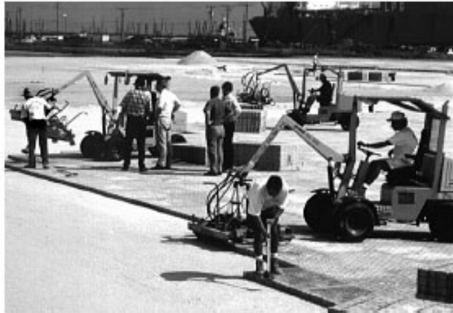
Figure 9. Mechanical installation equipment places concrete pavers rapidly.
