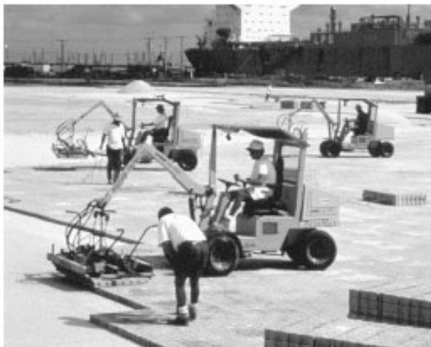
Figure 1. Mechanical installation equipment at Port of Tampa, Florida.
