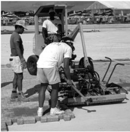
Figure 5. Motorized equipment with a hydraulic clamp.
