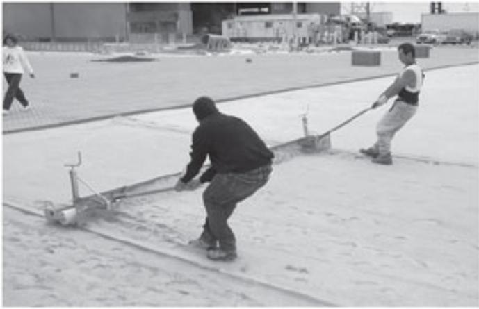
*Figure 4. A two-man hand pulled screed*
