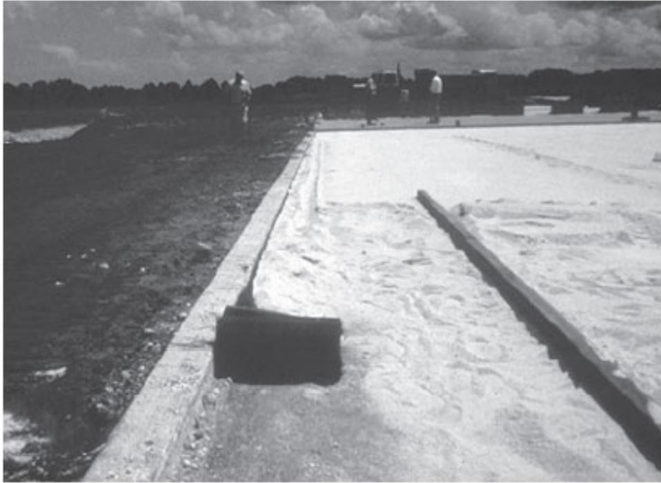
*Figure 7. Woven geotextile used to contain bedding sand from migrating laterally. Visit <[www.icpi.org](http://www.icpi.org)> for detail drawings.*
