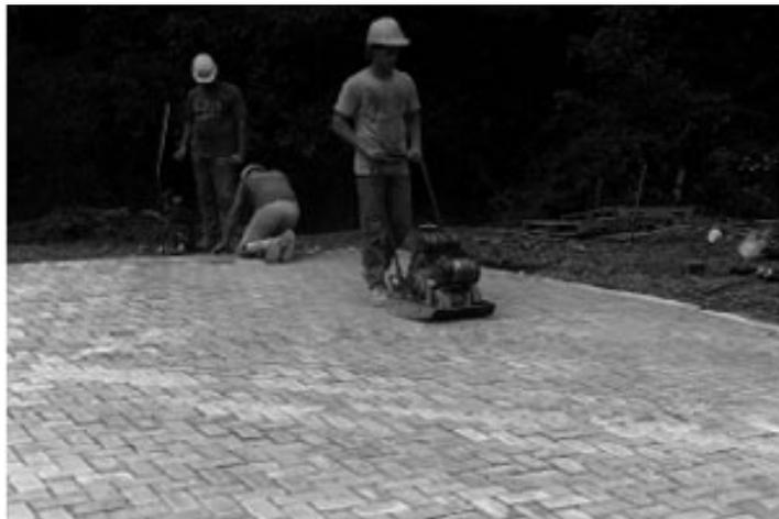
Figure 9. Compacting the pavers and bedding sand.
