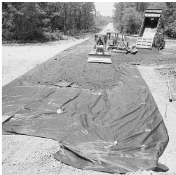
Figure 3. Application of the geotextile under aggregate base.
