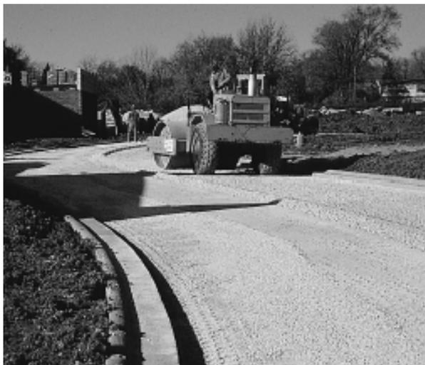
*Figure 4. Base compaction with a vibratory roller.*
