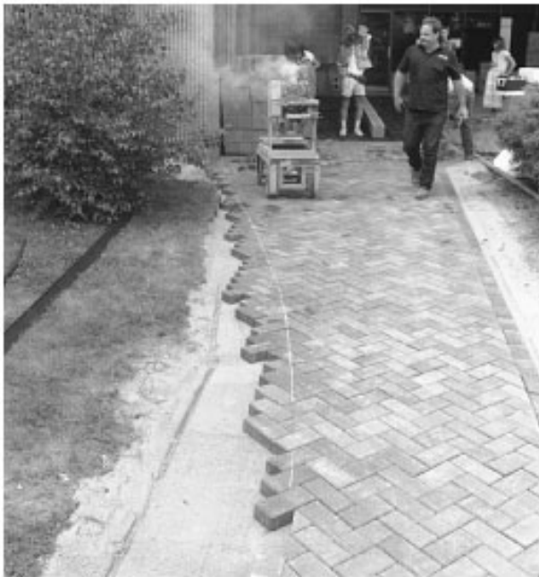
Figure 15. Saw cutting marked pavers on bedding sand. The cut pavers are carefully removed and edging is placed against the pavers and spiked in place.
