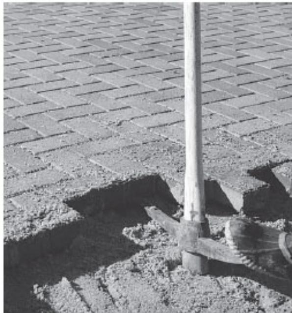
*Figure 6. Prying out the remaining pavers*
