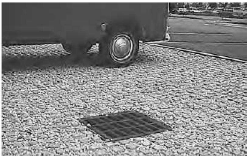
*Figure 18. Concrete grids with aggregate in the openings*
